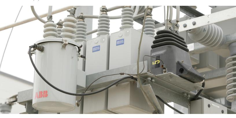
ABB's single-phase, pole-mounted "micropole" transformer designed for small, isolated load applications.
